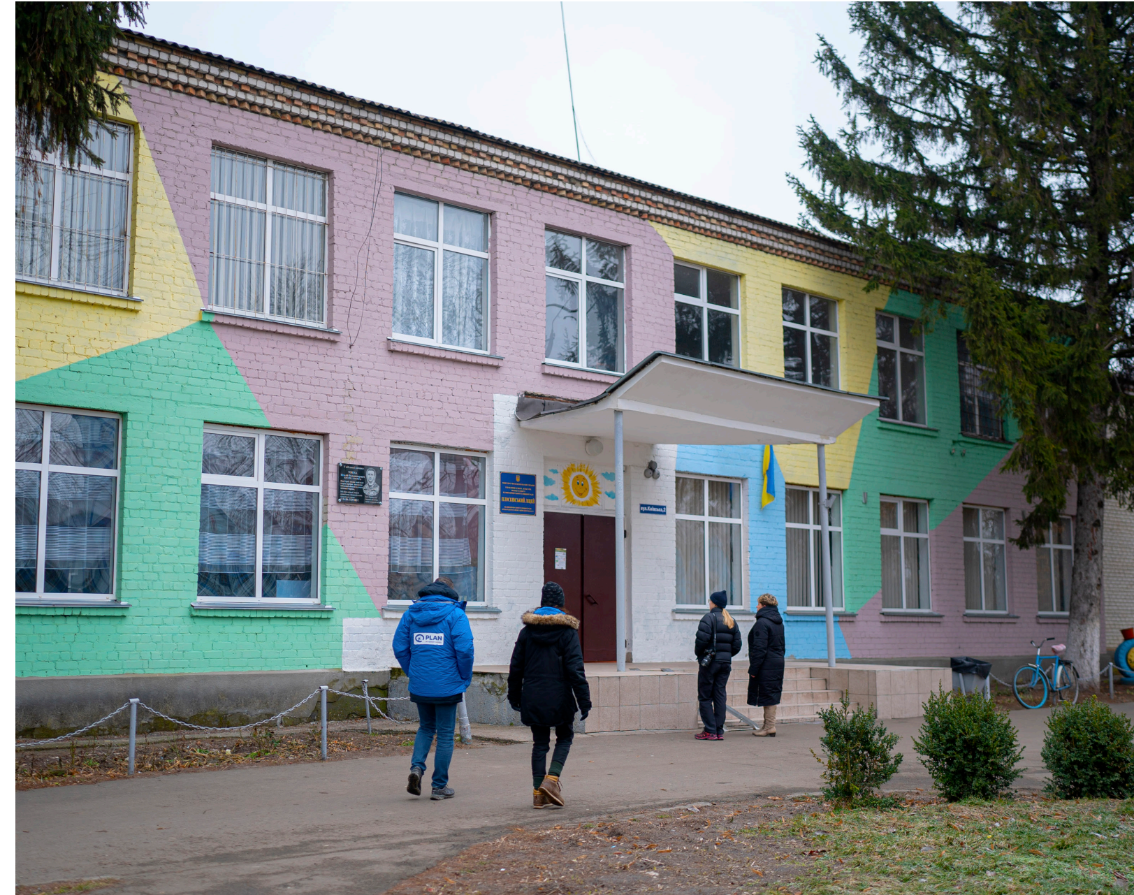
When part of this school building less than an hour’s drive from Kyiv was destroyed during fighting between Russian and Ukrainian forces, school staff and parents joined forces to rehabilitate it. The head teacher repainted the walls of the corridors herself, in bright colours, to lift the spirits of her pupils. Although sections of the school are still badly damaged, parts of it were able to be reopened to allow face-to-face learning – one of the few schools in the area to be able to welcome students back into the classroom.
